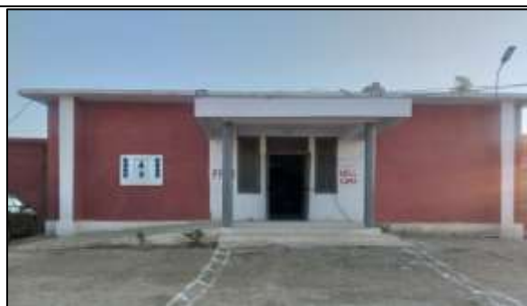
Figure 03 Existing Basic Health Unit in Rakhni, Front side
